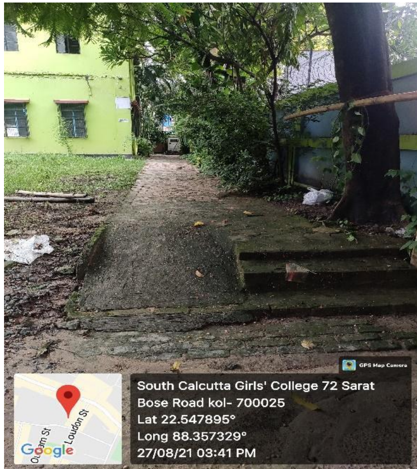
RAMP NEAR NORTH-WEST GATE
