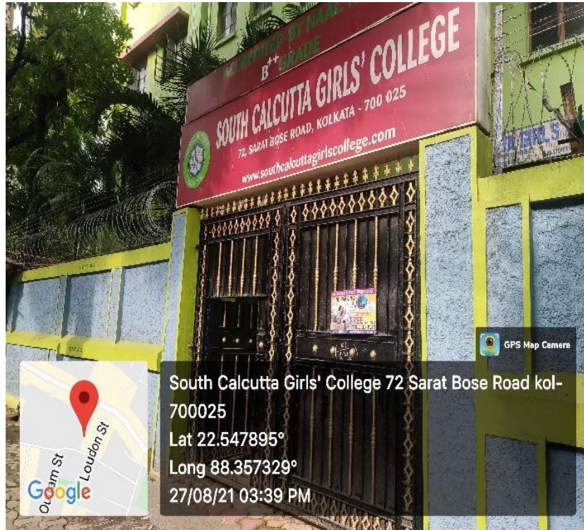
ONGOING RENOVATION OF GATE AND WALL
