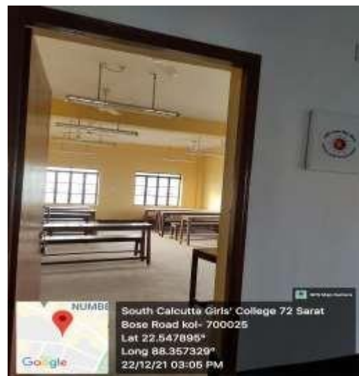
NEWLY ADDED CLASSROOM
