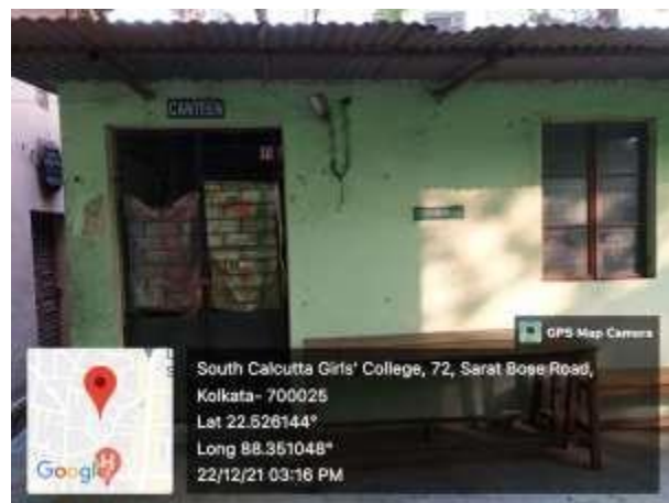
CANTEEN OUTSIDE THE MAIN BUILDING
